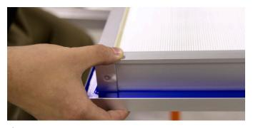
A) Using two people and being careful not to contact filter media raise the filter into place.
