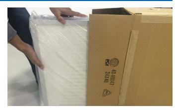
B) Remove filter from box being careful not to touch filter media.
