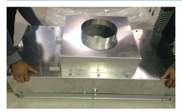
A) Place Krown Fan Filter Unit top cap assembly onto filter's gasketed flange/frame, being careful to not damage the filter media.
