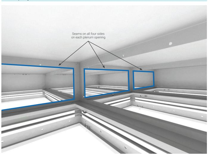
**Step 11:** Pull down the perimeter modules to tension the wires, and adjust the wire to minimize settling and moving of the plenum assembly once the damper and face are installed. Ensure that modules are tight to the adjacent ceiling system or drywall (if installed/applicable), and/or at the correct height and that there is no slack in the hanger wires.
