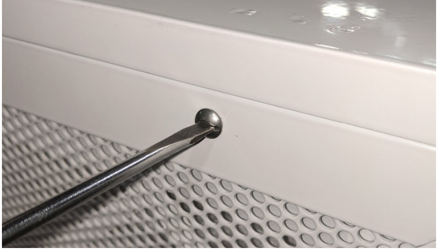
Diffuser Face with Quarter Turn Fasteners
